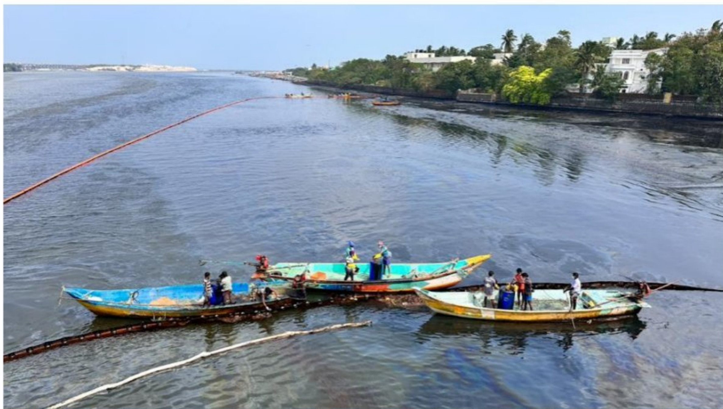
Figure 1: Oil spread near Ennore railway bridge
