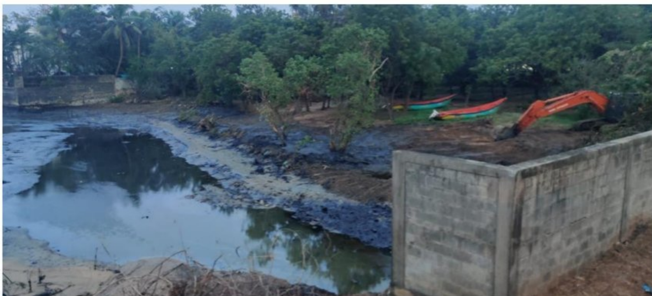
Figure 13: Earth moving machinery at the oil spill site
